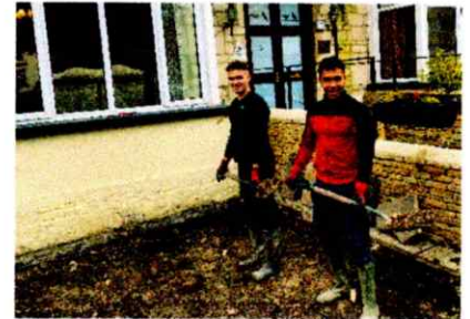
Landscape gardeners working hard!
